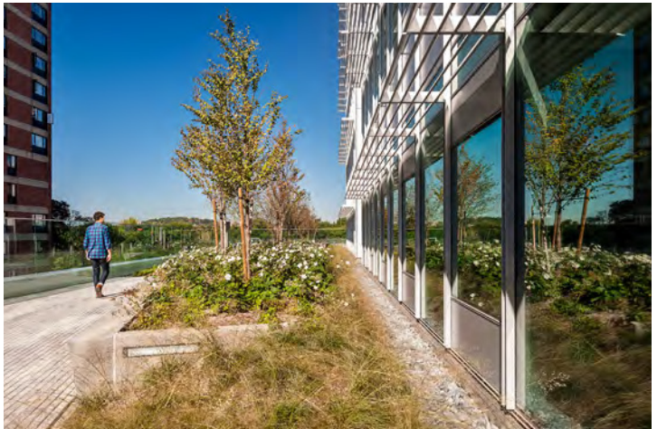
Hale Building for Transformative Medicine
